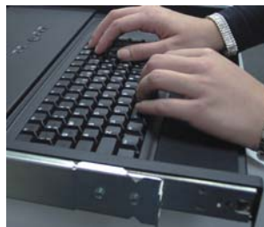
Access SUN servers directly from the rack
